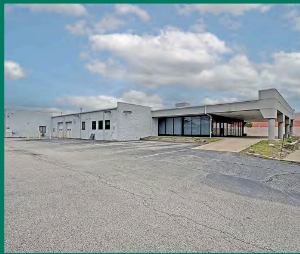
REAR (2) 10'x10' OVERHEAD DOORS
