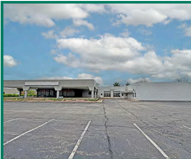
FRONT (2) 10'x10' OVERHEAD DOORS
